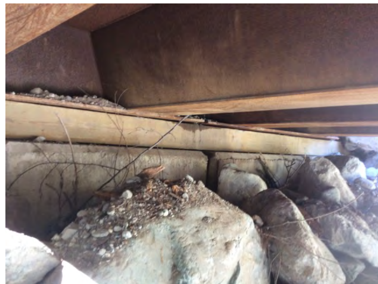
Left Bank Abutment when facing downstream
