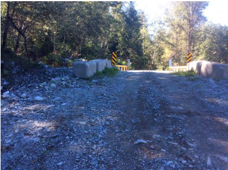
Approach from Right Bank when facing downstream
