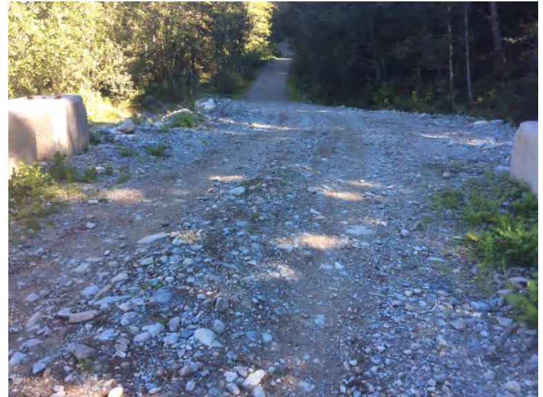
Approach from Right Bank when facing downstream
