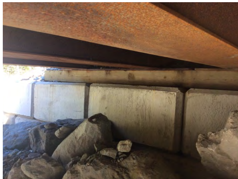
Right Bank Abutment when facing downstream
