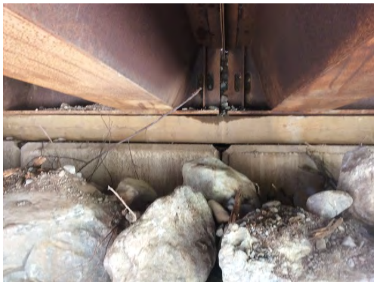
Left Bank Abutment when facing downstream
