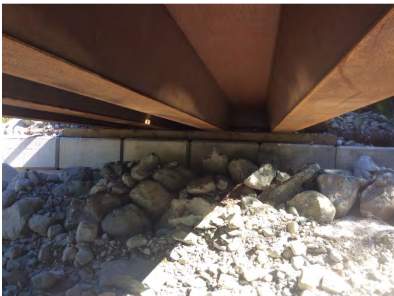
Right Bank Abutment when facing downstream
